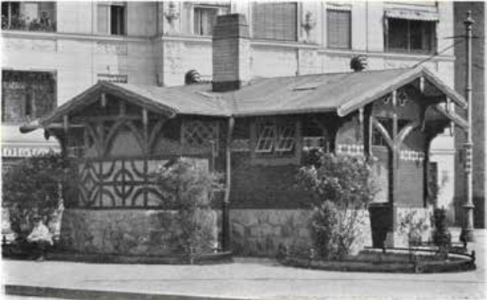
View from the Kantstraße
