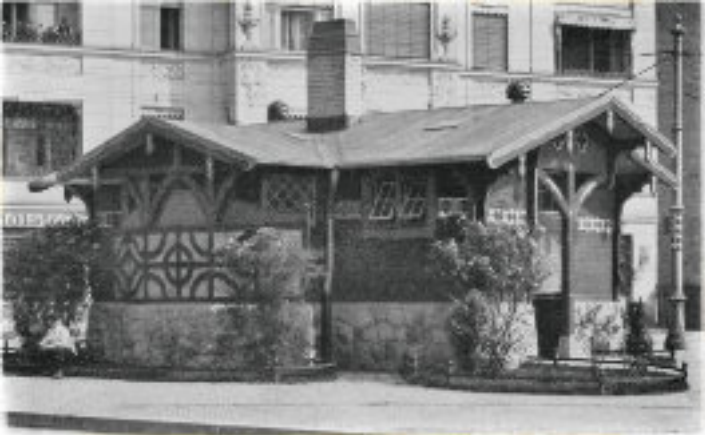
View from the Kantstraße
